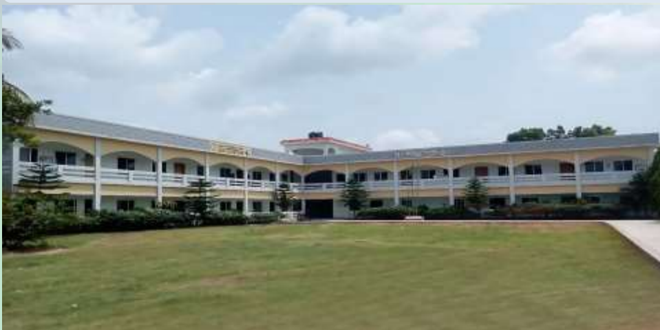
2 STORIED MADRASAH BUILDING AT MADARIPUR
