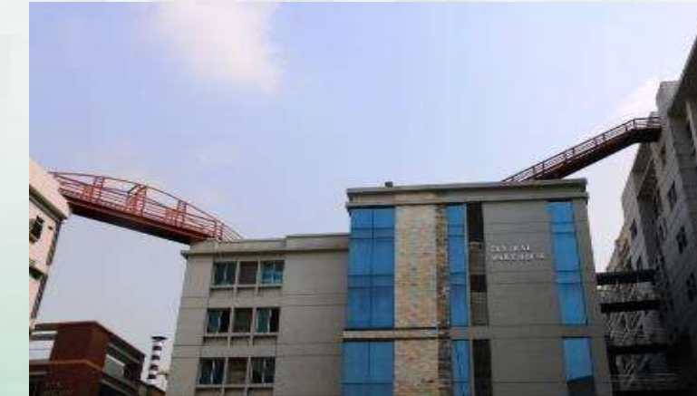
BUILDING TO BUILDING CONNECTING BRIDGE
