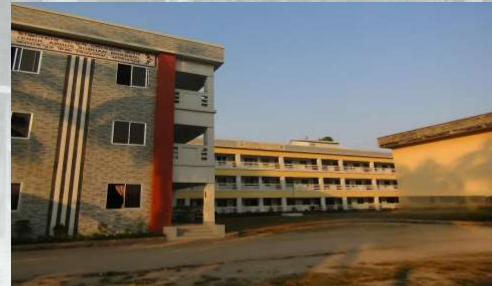
3 STORIED SCHOOL BUILDING AT KANAIPUR, FARIDPUR
