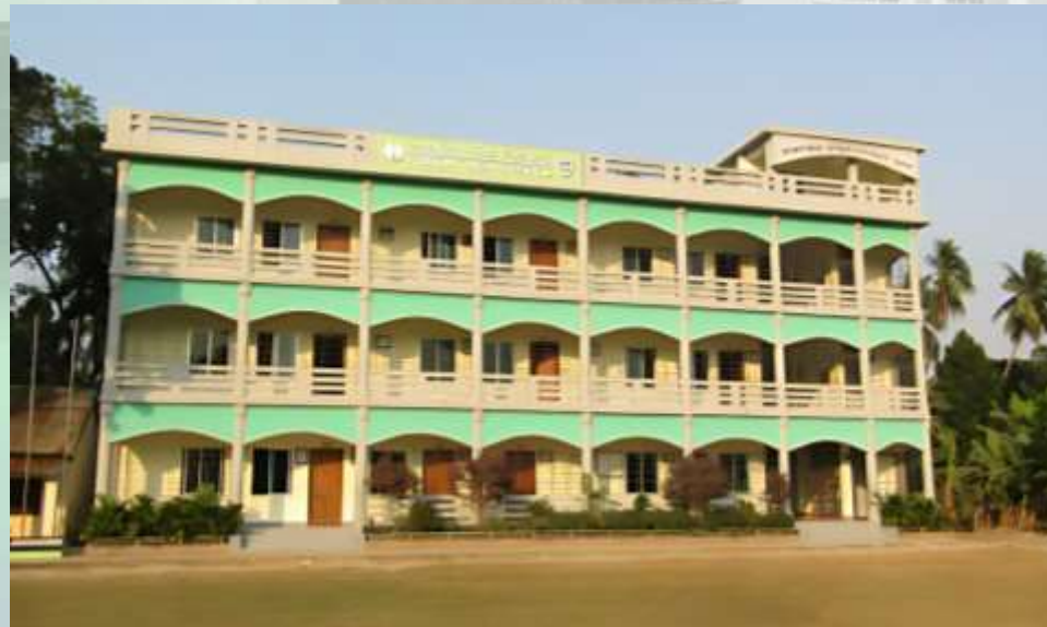
3 STORIED SCHOOL BUILDING AT PURDIA, FARIDPUR
